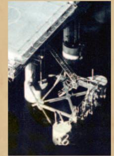
Once Mr. Charlie was towed to the drill site, the pontoons were lowered and then the barge, pontoons and structural legs were flooded with seawater until negative buoyancy was achieved. Once the flat-bottomed hull settled on the seafloor, "making hole" began.
